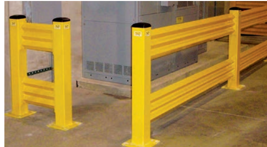
Guarding electrical panels
