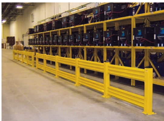
Guarding battery racks
